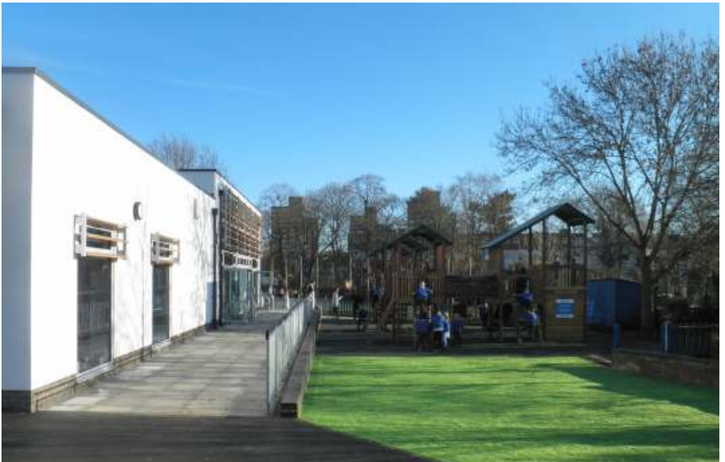
The back of the school, now complete
